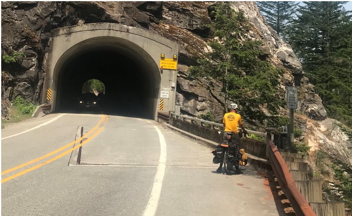
Figure 16. Tunnel in Washington State, USA
